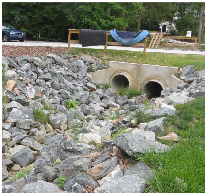
Repaired drainage pipes
