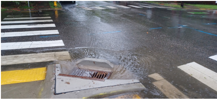
Stormwater Drain on East Franklin Street
