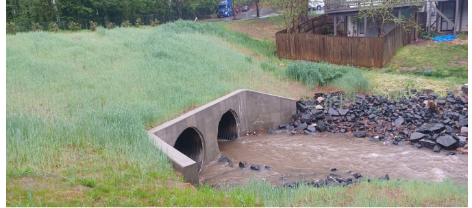
Burgess Court Stormwater Headwall
