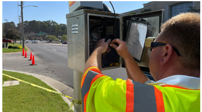
Stormwater staff installing a rain gauge on Glenwood Avenue
