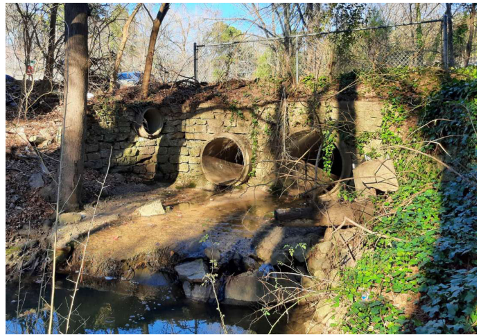
Stormwater pipes at Dacian Drive
