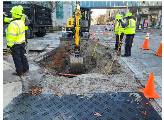
Stormwater staff repairing stormwater pipe on West Jones Street
