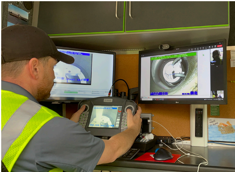
Stormwater staff performing a pipe repair
